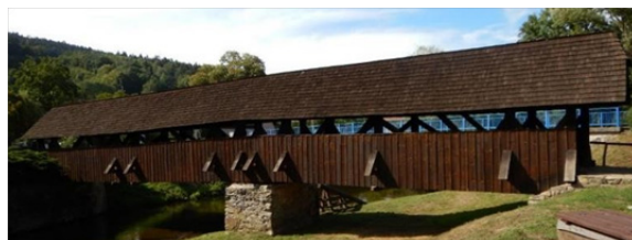
Fig. 1: Bridge Černvít in the ČR (Bak et al. 2012).
