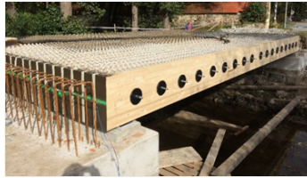
Fig. 1: First transversely prestressed bridge in the Czech Republic.
