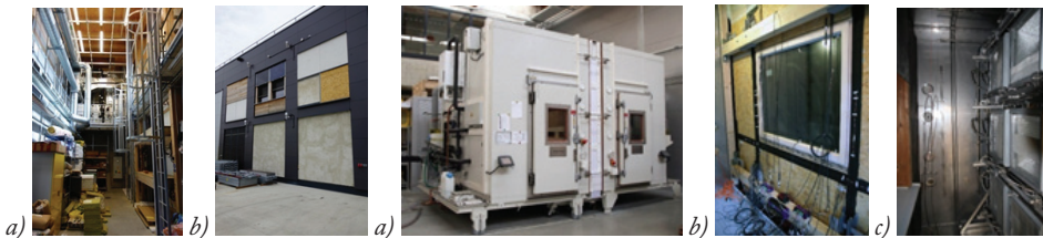
Fig. 1: Climatic room a) wooden interior of climatic room with HVAC systems, b) experimental façade with six “windows” for installation of fragments of building constructions.
