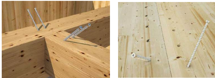
Fig. 1: The engineering application of self-tapping screw.
