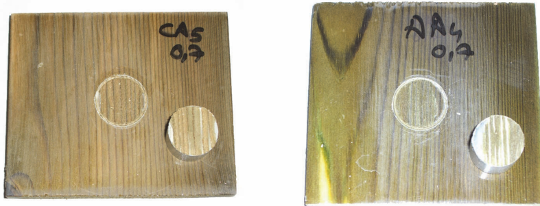
Fig. 2: Varnish flaking and wood failures on pine wood surface
