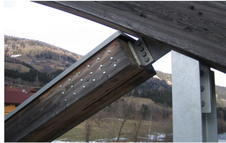
Fig. 2: Two shear plane connection steel-timber / metal dowels and bolts. Fig. 3: Two shear plane connection steel-timber / metal dowels.
