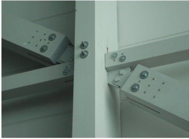
Fig. 2: Two shear plane connection steel-timber / metal dowels and bolts. Fig. 3: Two shear plane connection steel-timber / metal dowels.
