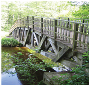
Fig. 1: Investigated bridge (photo: Lerche 2010).
