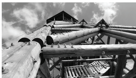
Fig. 1: Watchtower near Lázně Bohdaneč – round timber bolted joints with slotted-in plates.
