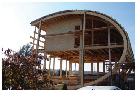
Fig. 12: Load-carrying structure made from curved segments.
