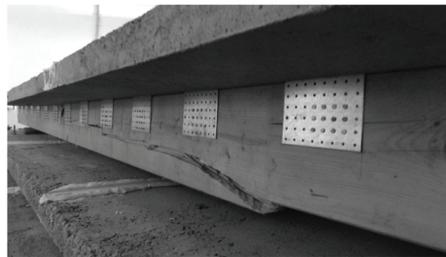
Fig. 12: Damage of timber beam along grains.
