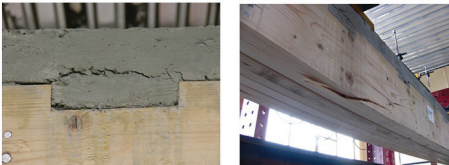
Fig. 7: Failure modes of the vertically laminated timber-concrete composite beam.
