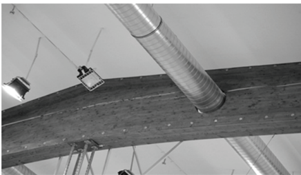
Fig. 5: The effect of sloping grain in tapered beam (unheated indoor environment).
