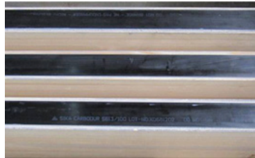
Fig. 5: Reinforced glulam beams (Group B).
