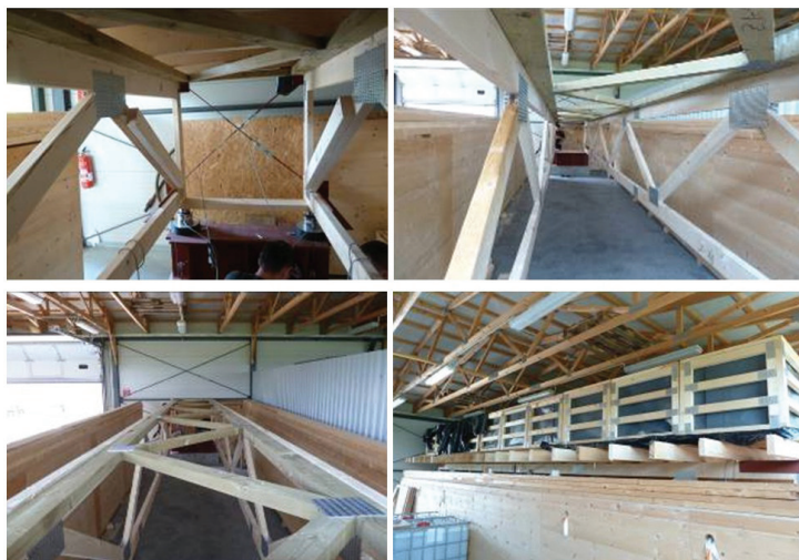
Fig. 1: Investigated samples and platform with containers at the top of trusses.
