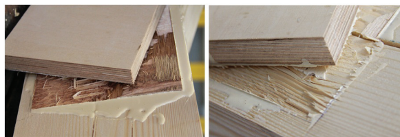
Fig. 8, 9: Damage in timber plywood veneer and timber element.
